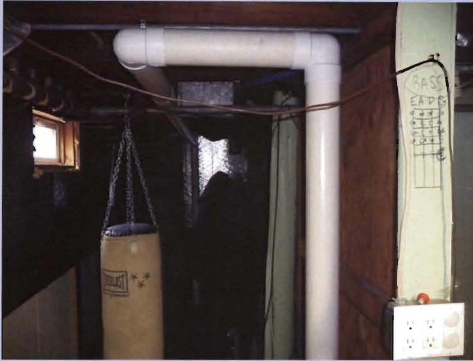
Showing how the two vapor extraction locations are plumbed together to the outside.
