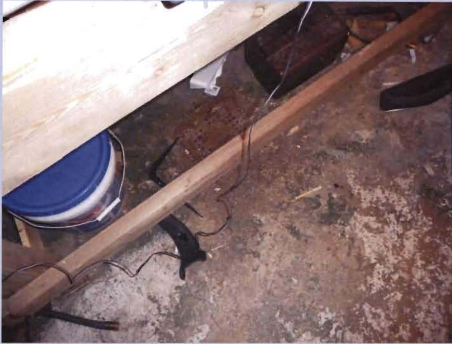
Shows the presence of floor drains in the basements which would act as conduits for vapor to enter the buildings.
