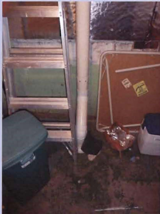
Showing the vapor depressurization system location directly adjacent to the wall. Notice the poor condition of the wall and the concrete floor.
