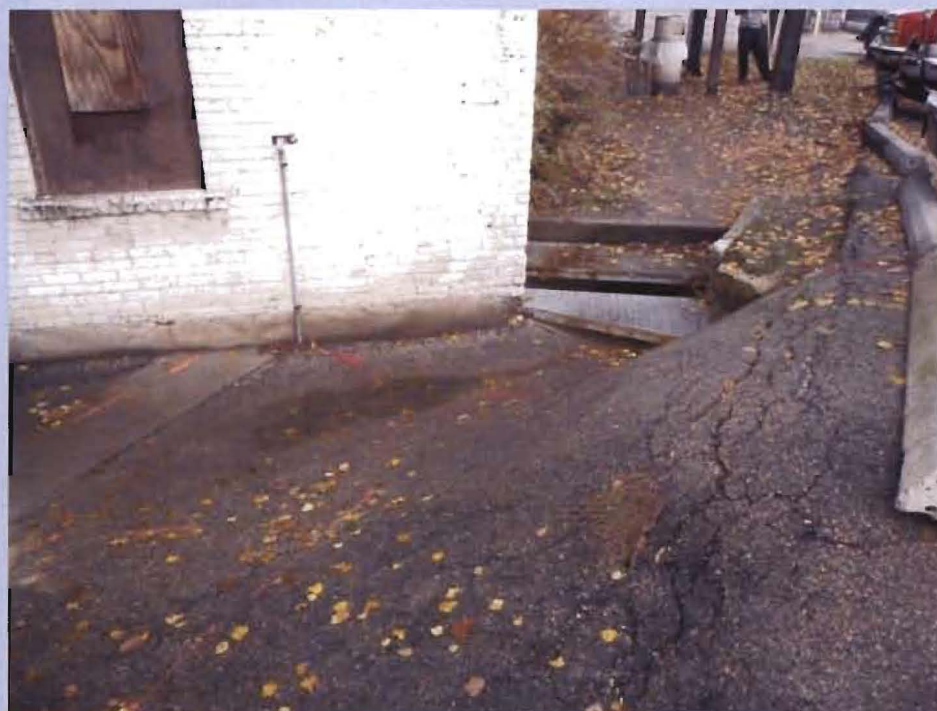
Showing the drainage from the above ground storage tank area flows to a subsurface drain heading towards the northern part of Madison-Kipp property.
