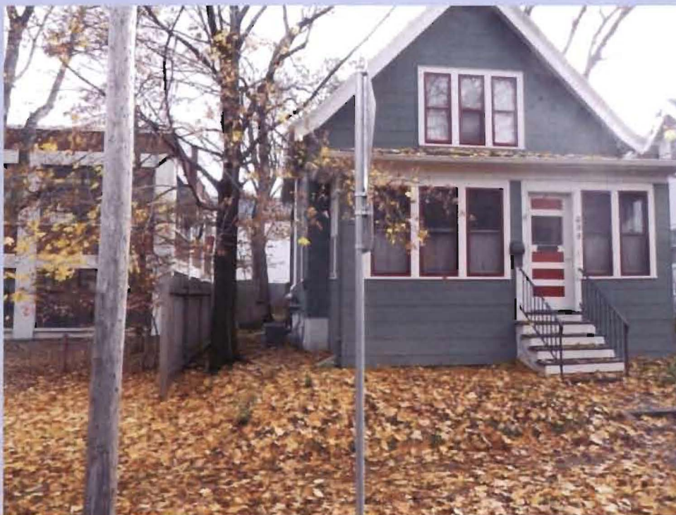
Showing the home at 233 Waubesa Street. Note the vapor depressurization system on the left hand side of the home. Also note the immediate proximity of the Madison Kipp vents located on the Madison-Kipp property.
