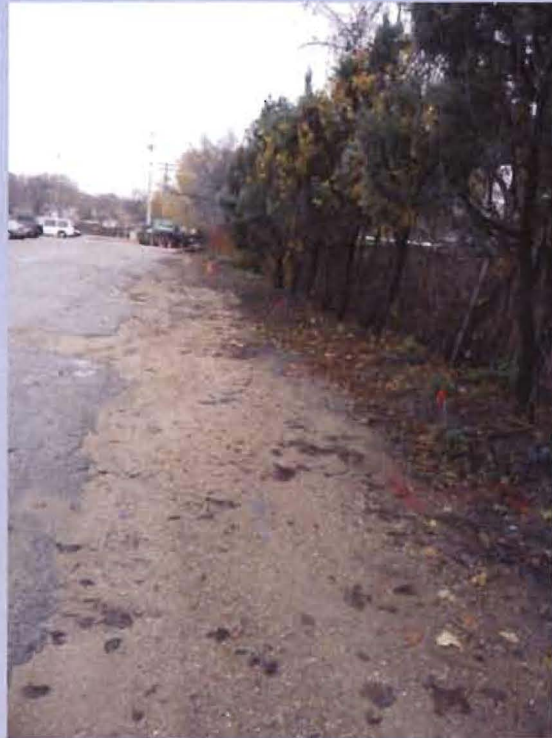
Looking towards the northeastern side of the Madison-Kipp parking lot showing how the drainage is to the east into the neighboring family properties.
