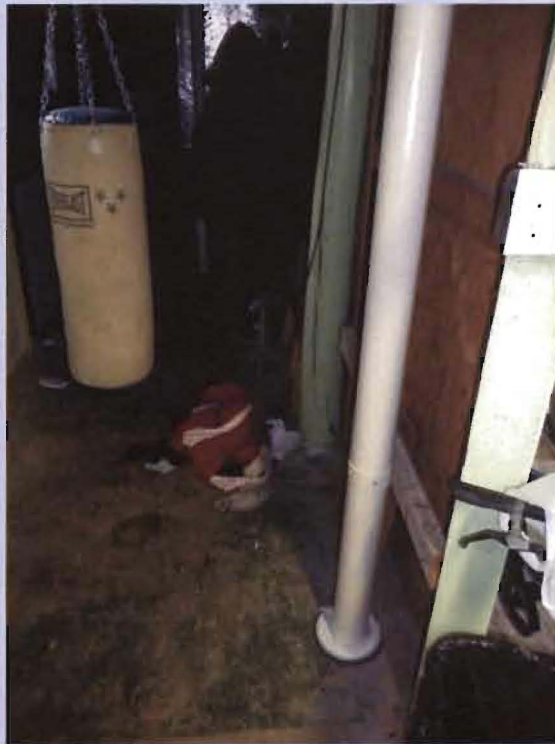
Showing a second location for the depressurization system in a clients home.
