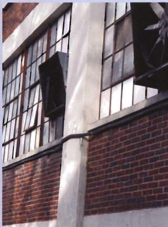
Close-up of the window vents showing the buildup of various petroleum tars caked around the vents.
