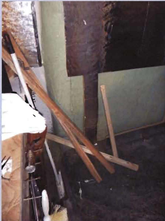
Showing the condition of the concrete in the basement. The cracks in the wall would allow contaminated vapors to enter the basement.
