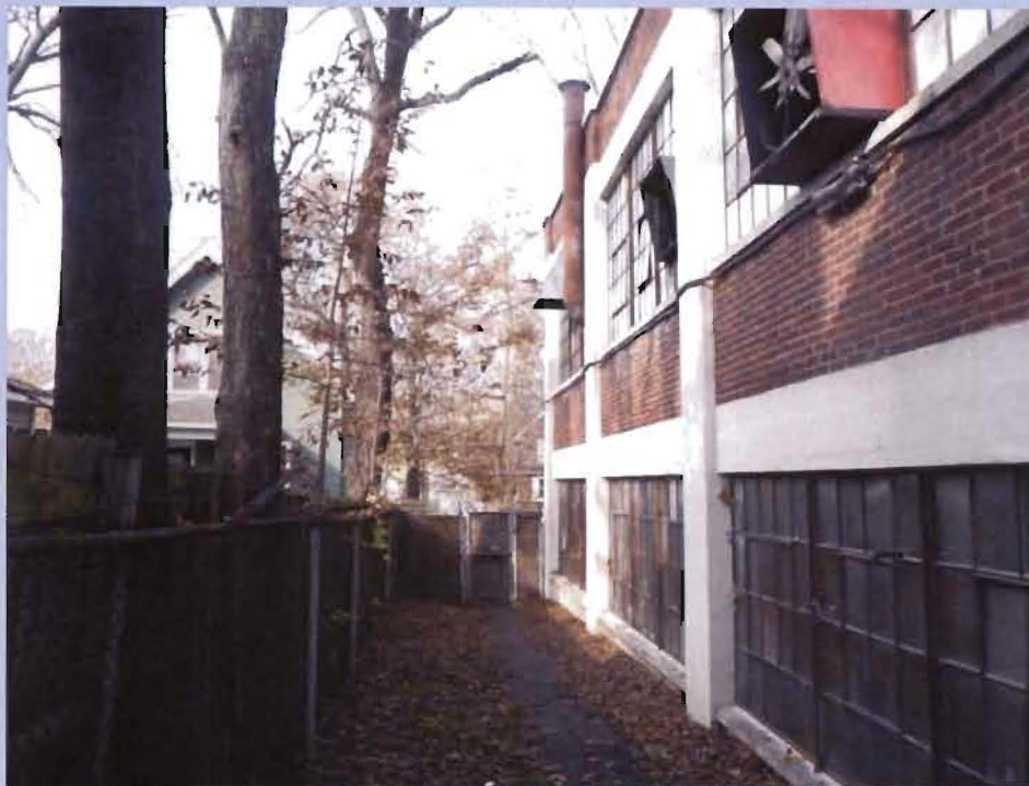
Looking due west at the edge of the Madison-Kipp facility. Note that the property to the left would be 233 Waubesa Street. Note the three vents projecting through the windows and the one vertical vent.
