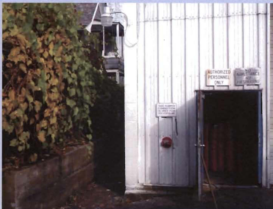
Looking north from the southwestern parking lot. Note narrow passage way between Madison-Kipp property and home at approximately 269 Waubesa Street.
