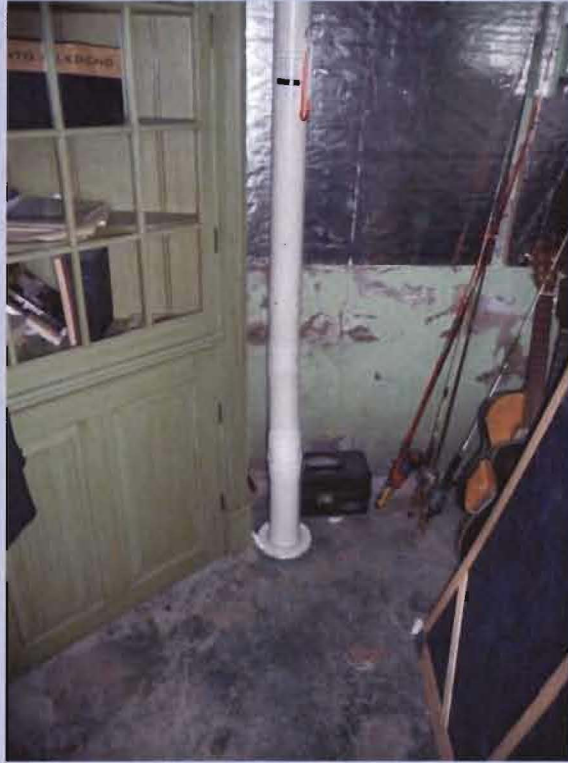
Showing a vapor extraction system. Note the condition of the concrete wall in the background and the condition of the floor.
