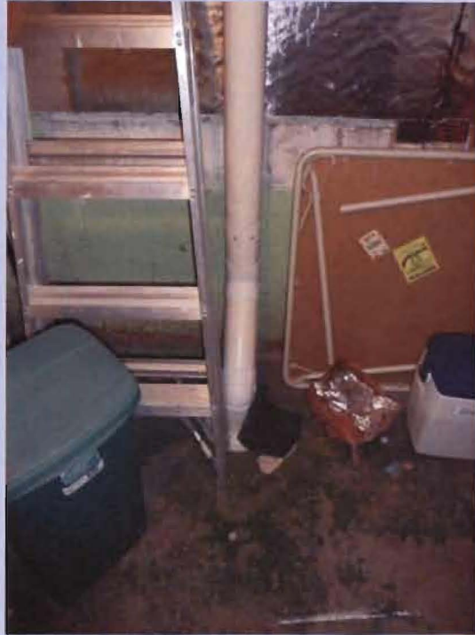
Showing the vapor depressurization system location directly adjacent to the wall. Notice the poor condition of the wall and concrete floor.
