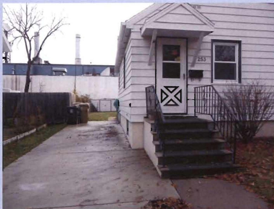
Shows the huge roof stacks associated with the Madison-Kipp facility directly adjacent to the backyards of homes.
