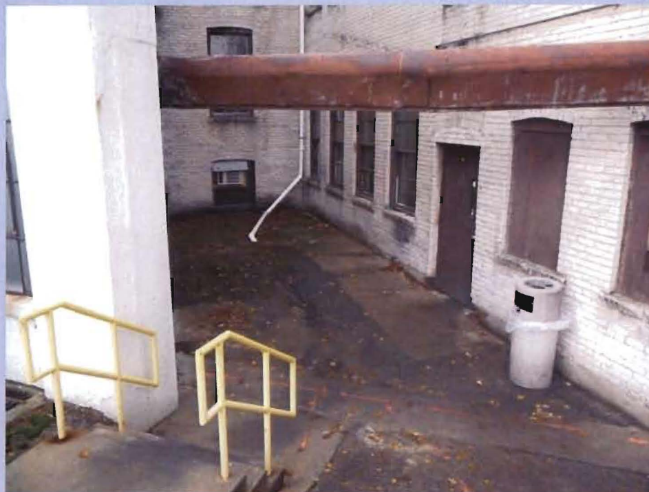
Showing the location of the above ground PCE storage tank. Note, no indication of soil samples taken. Note that the surface flow is towards the front of the picture.
