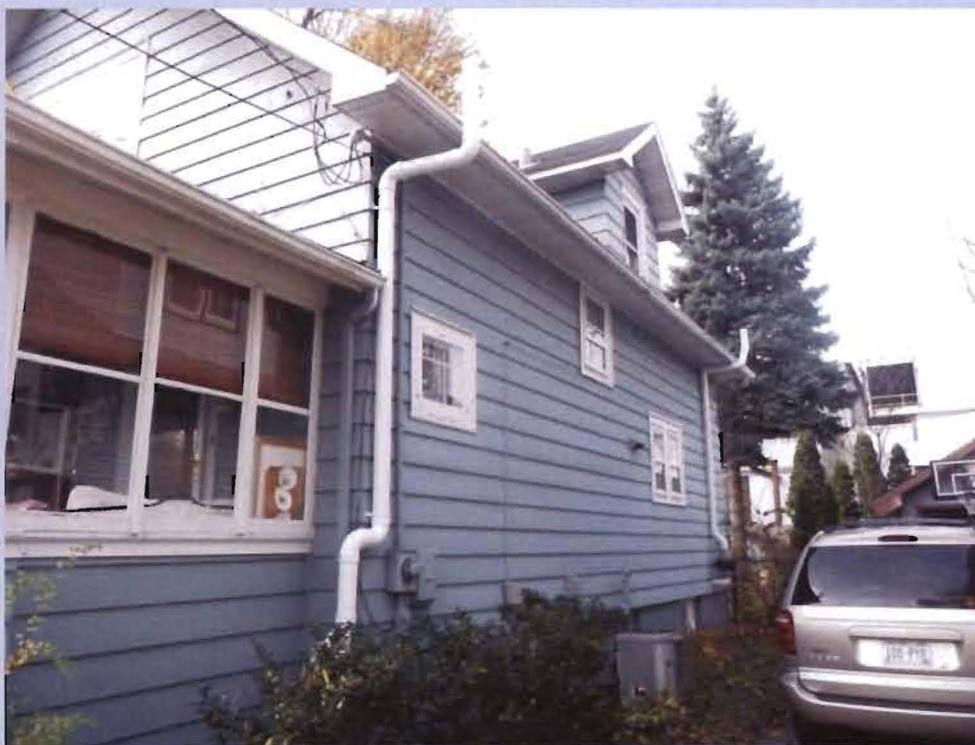
Showing two separate depressurization systems on the north side of this home on Marquette Street. Note the location of the 2 vapor depressurization systems relative to the 2 rain gutter downspouts.
