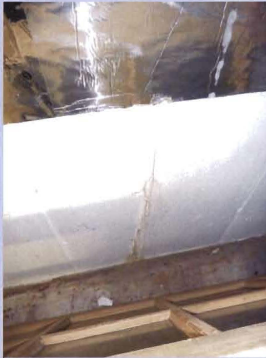
Showing the cracks in the concrete wall and the seepage of moisture through the cracks.
