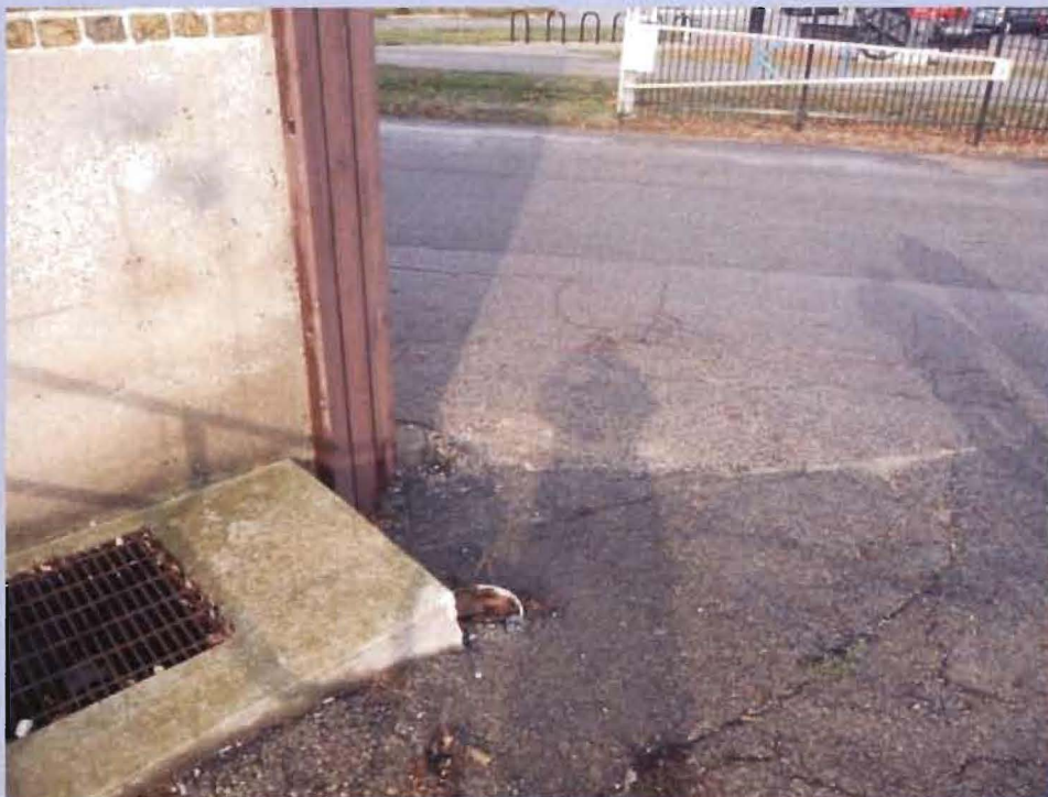
Shows a drainage grate down gradient from the above ground storage area. The subsurface sewer then turns towards the north east towards the bicycle path noted in the top of the picture
