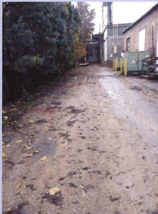
Looking south and noting how the drainage is to the east into the neighboring properties.
